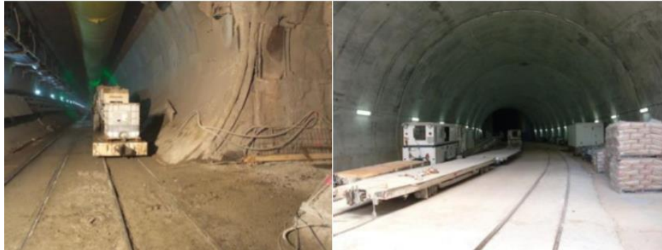
Figure 1 ACCIONA platform wagons (source ACCIONA)
