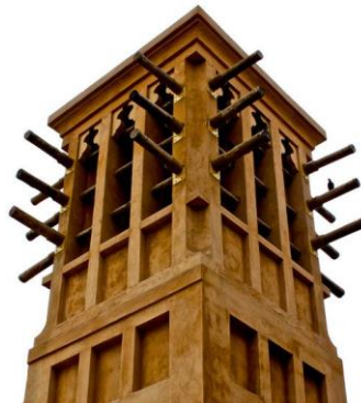
Figure 1. Ventilation ducts - traditional Arabic architectural signs
