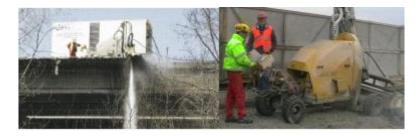
Fig. 3. Hydrodemolition of bridge plates by Conjet robots
