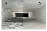
Figure 4. Air conditioning duct status A) dirty; B) clean
